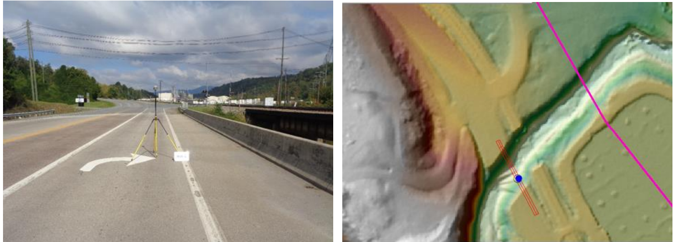
Figure 13. NVA-06 is located on a bridge deck which has been removed from the DEM, which can be seen on the right. The blue point represents NVA-06 on the DEM.
