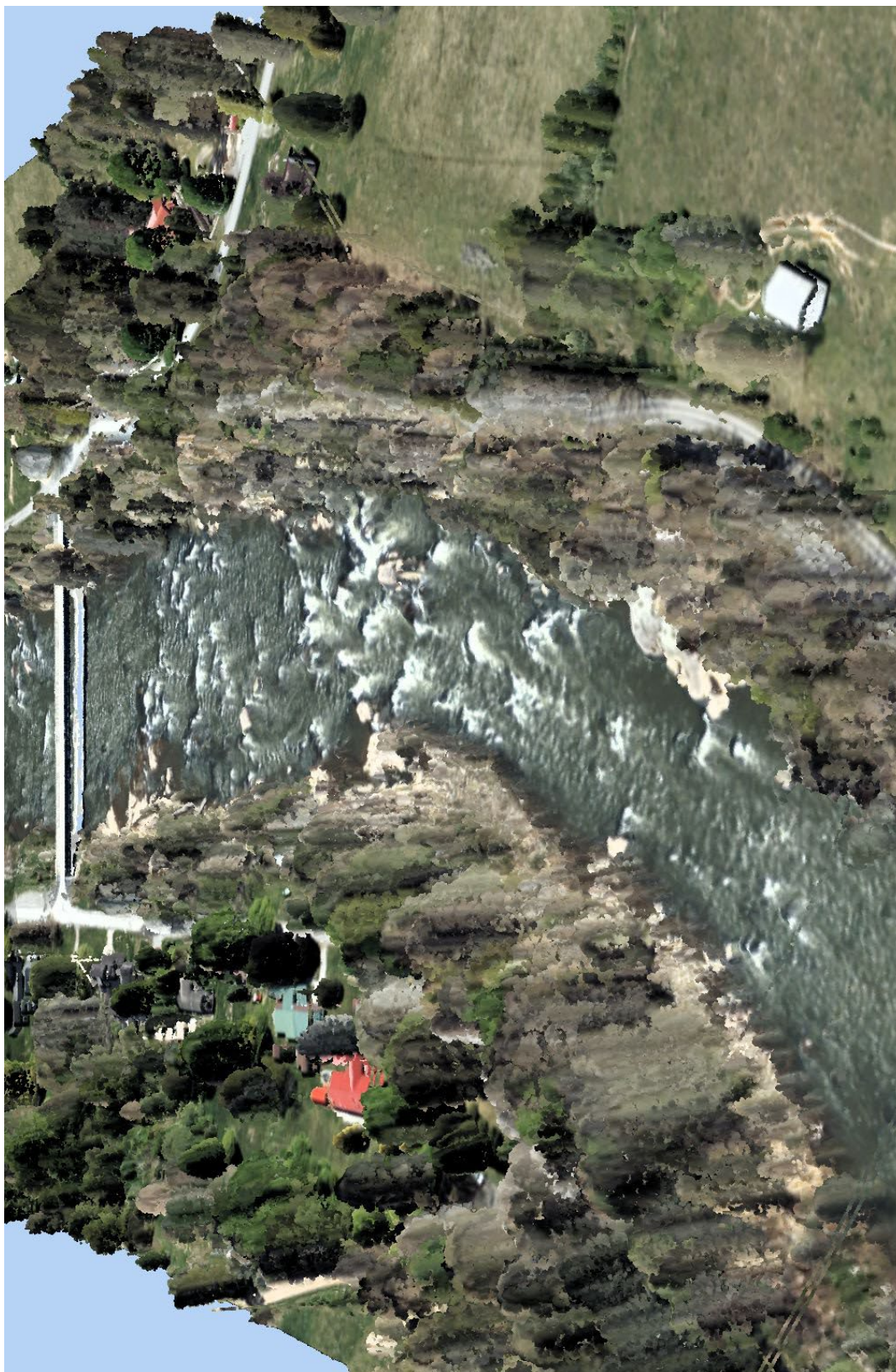
Figure 46: View looking southwest at the North River Road Bridge near Arden Falls on the Tygart Valley River in the NOAA Appalachia project area. The image was created from the lidar bare earth model overlaid with the above-ground point cloud and orthoimagery.
