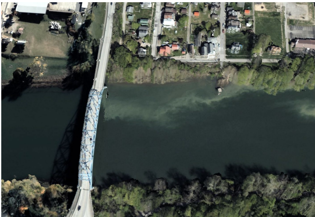
Figure 48: View looking east at the Historic Point Marion Iron Bridge on the Monongahela River in the NOAA Appalachia project area. The image was created from the lidar bare earth model overlaid with the above-ground point cloud and orthoimagery.
