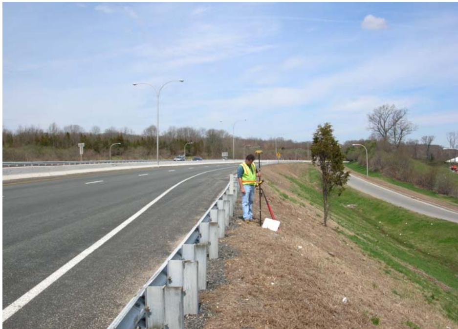
NO. 14 4/26/07 PT. 2306 - LOOKING NORTH
