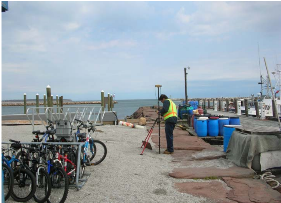
NO. 12 4/30/07 PT. 2405 - LOOKING NORTHEAST
