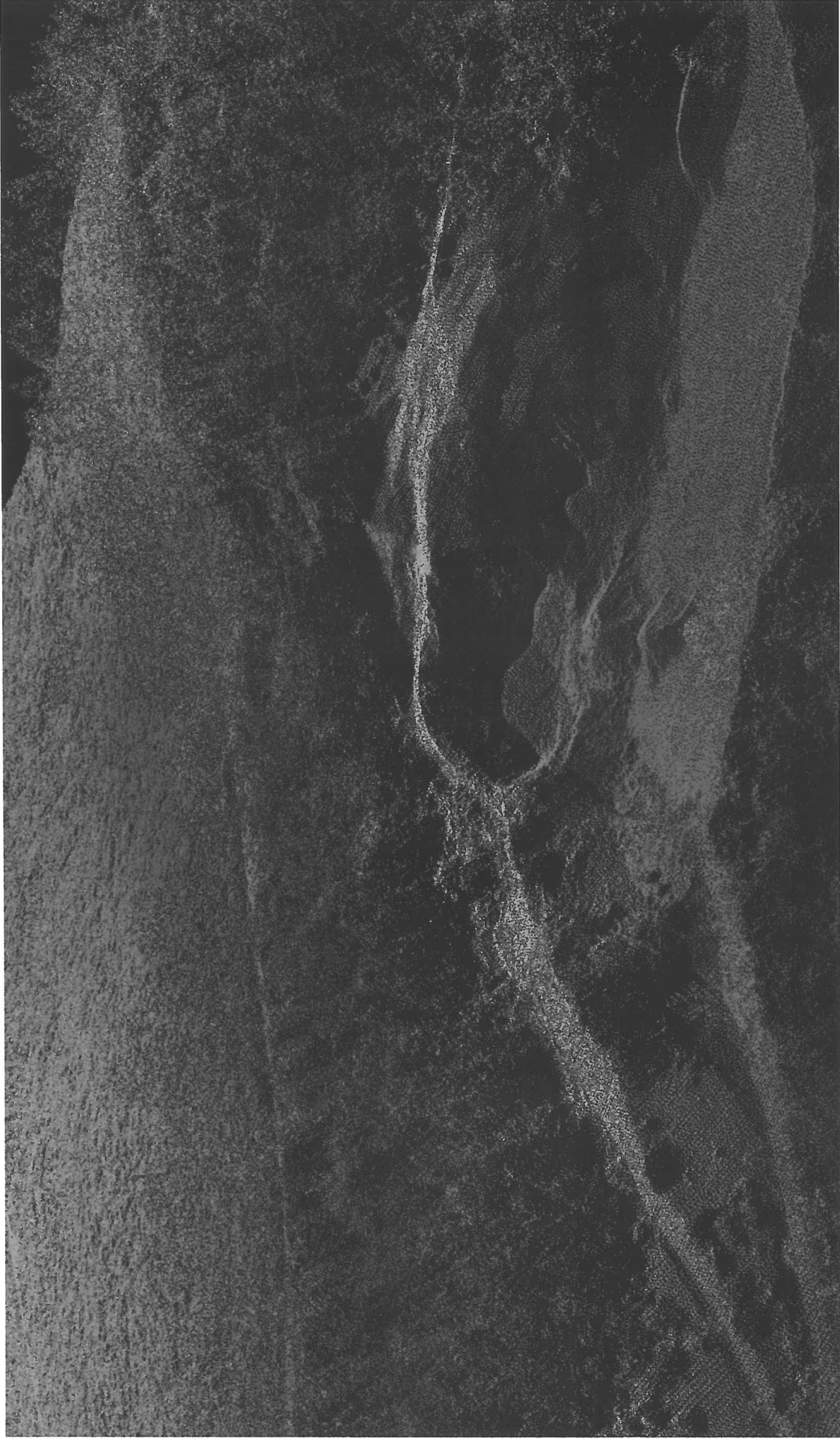
Figure 10. View of construction area created from LiDAR point cloud colored by height.
